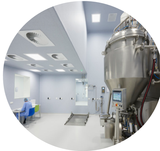
Cleanrooms and labs
